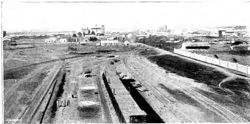
SOUTH-EASTERN ENTRANCE TO CENTRAL ARGENTINE RAILWAY, ROSARIO.
